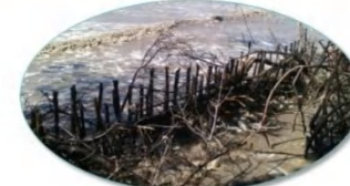
Construction of palisades
